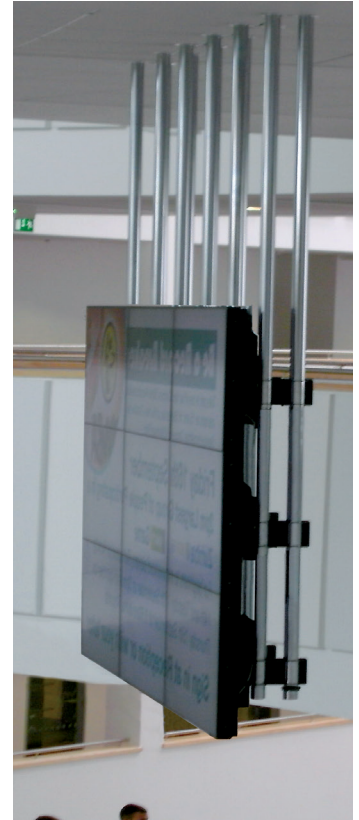
3x3x46" Ceiling Suspended video wall, Cheshire University
